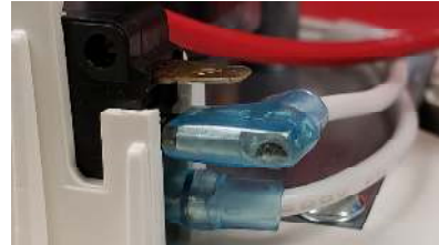
Fig. 3: High level float contacts in N.O. position
