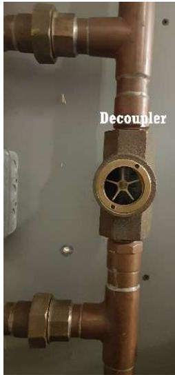
I have hydronic training boards that have a P-S connection with a sight flow indicator in the decoupler (common) pipe, as shown to the left. By manipulating the primary and/or secondary flows, the decoupler flow can be made to go in either direction. I always enjoy some of the 'Aha!' moments when people see that paddlewheel stop and go the other way.
